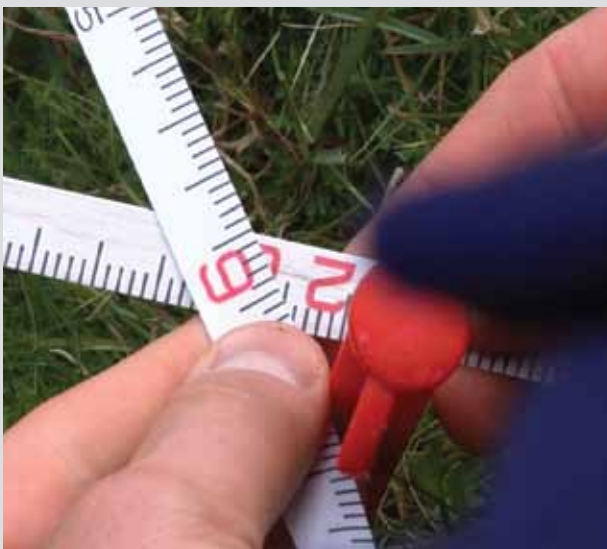
Pulling two tape measures tight to establish one corner of a 3:4:5 triangle.
